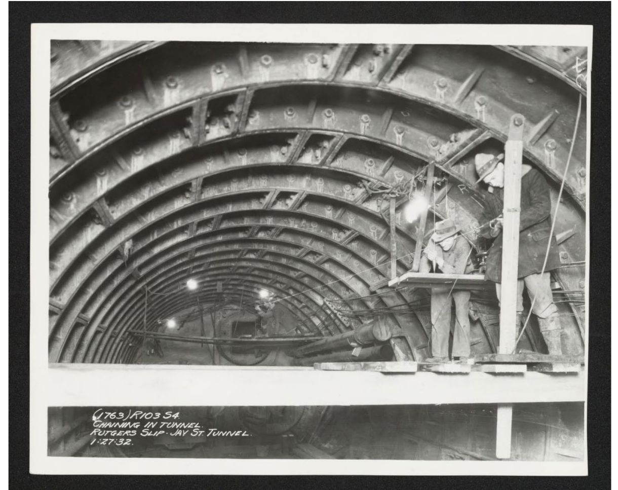
The tunnel under construction
