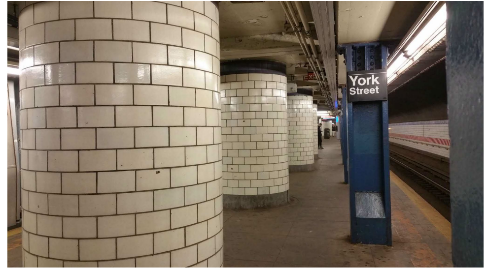
Manhattan Bridge underpinning piers on the platform
